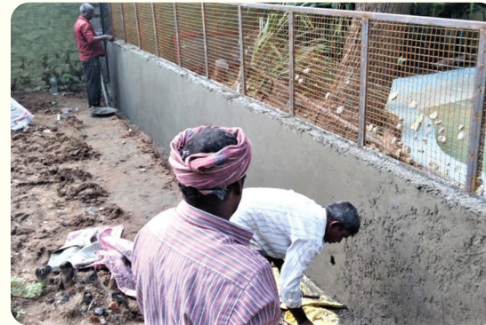
g) Reconstruction of Damaged Wall between Gharial and Mugger Crocodile
